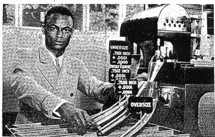
Claude Harvard, mechanical genius of The Ford Motor Company, demonstrating remarkable measuring machine, accurate to one-millionth of an inch, which he helped develop and build
